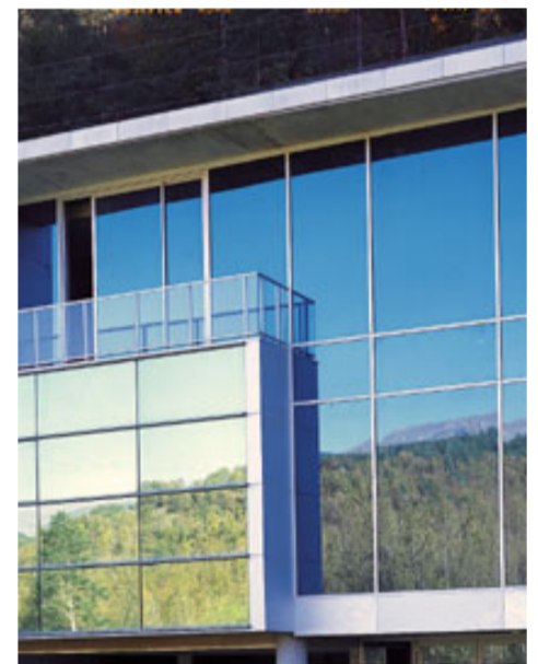
Detail of the change in geometry in the main façade
