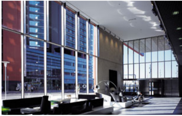
The hall is glazed with a Mecano curtain wall and traditional grid
