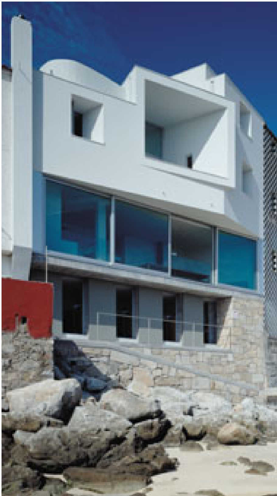
Stone, concrete, glass white rough plastering are the finishes that determine the façade make-up
