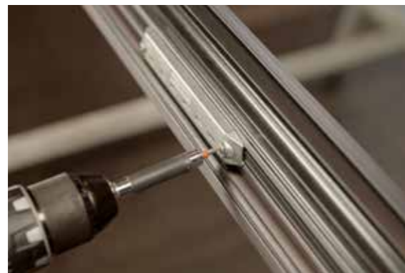
Direct punching of the tie rod
